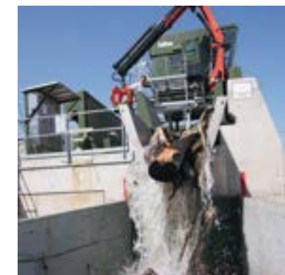
Debris sluice way
