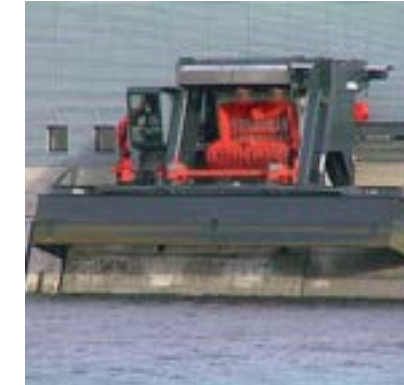
Stop log handling - Rope Type
