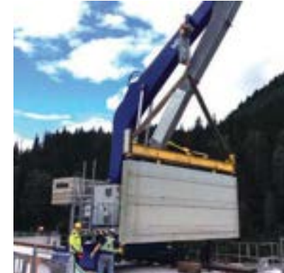
Stop log handling - Hydraulic Type
