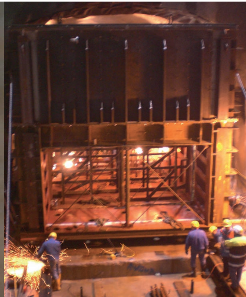
Assembling draft tube gate
