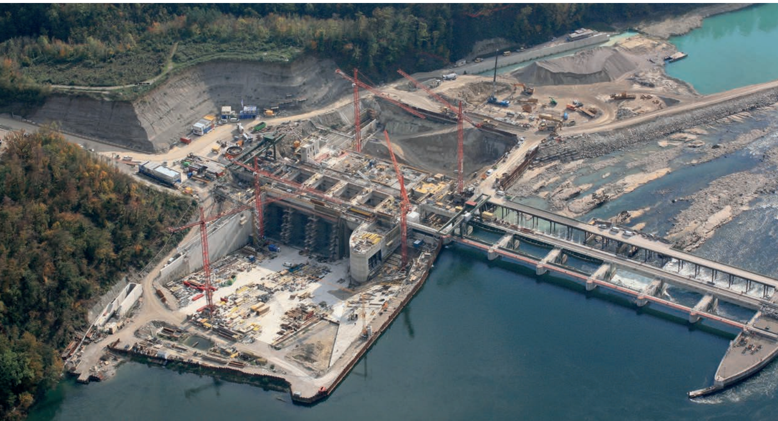
Construction pit before flooding in 2010
